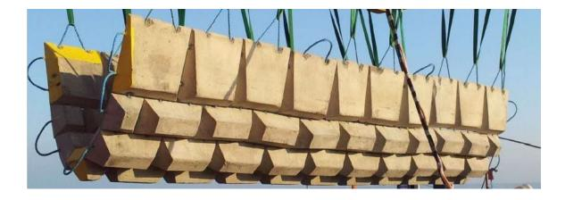
Figure 10-8. Example of Concrete Cable Protection Mattresses
