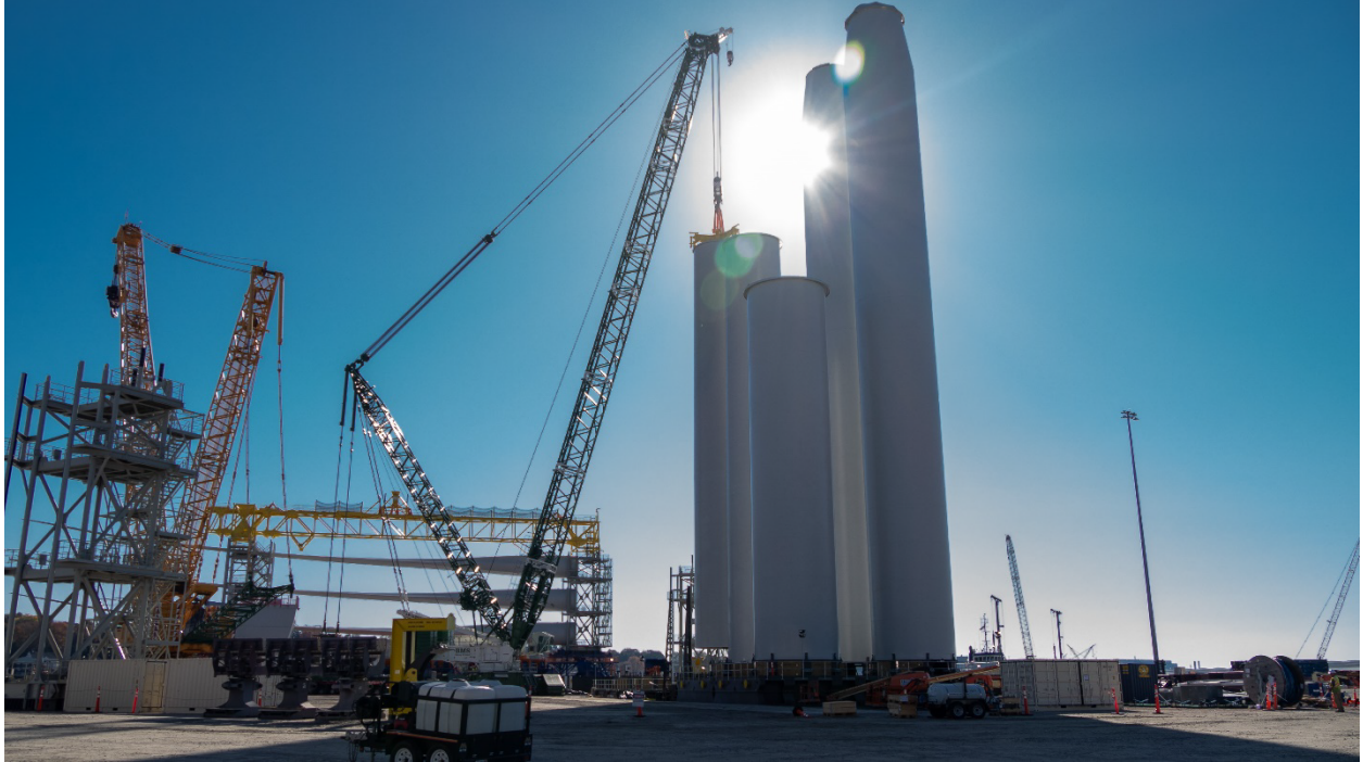
Figure 10.6: Tower Section in Pre-assembly at New London State Pier (South Fork Wind, 2023)
