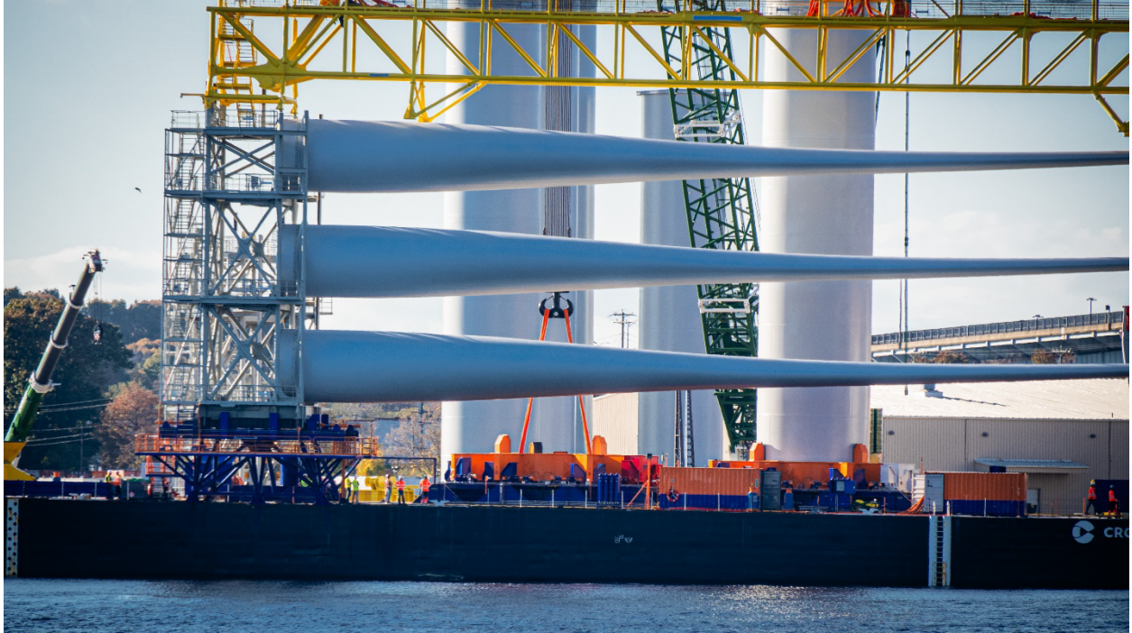
Figure 10.8: WTC Components Being Loaded Out at New London State Pier (South Fork Wind, 2023)
